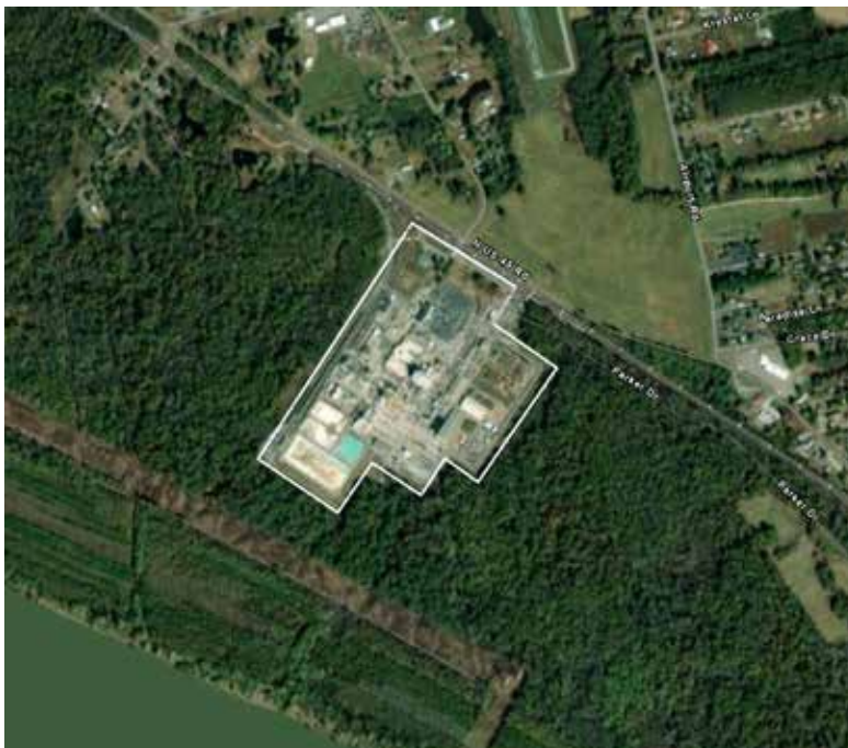
Honeywell Inc.'s Metropolis Works uranium-conversion facility, on the banks of the Ohio River.
