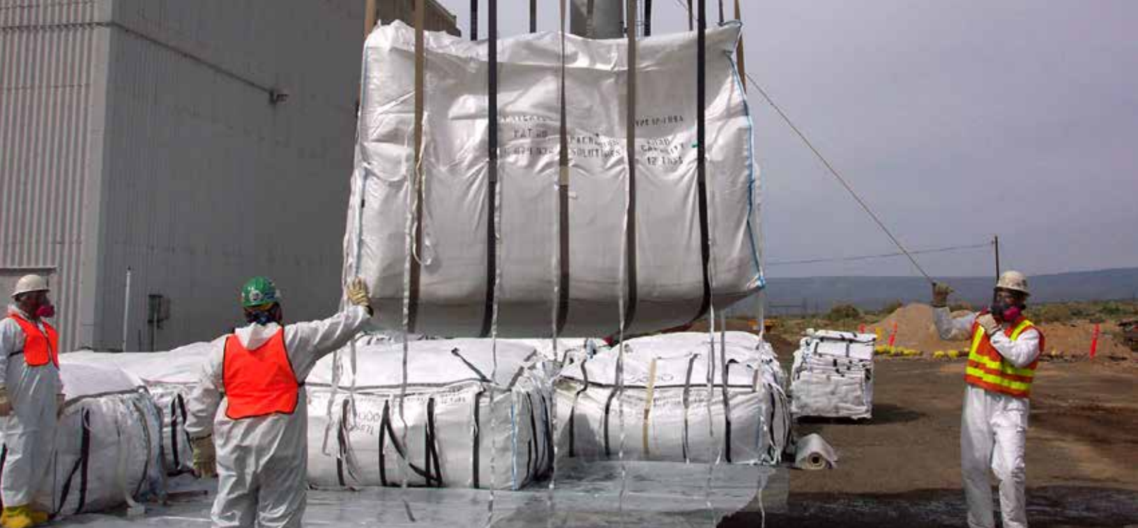
An example of SuperSaks, which are often used to package waste for transport to the White Mesa Mill. U.S. DEPARTMENT OF ENERGY
