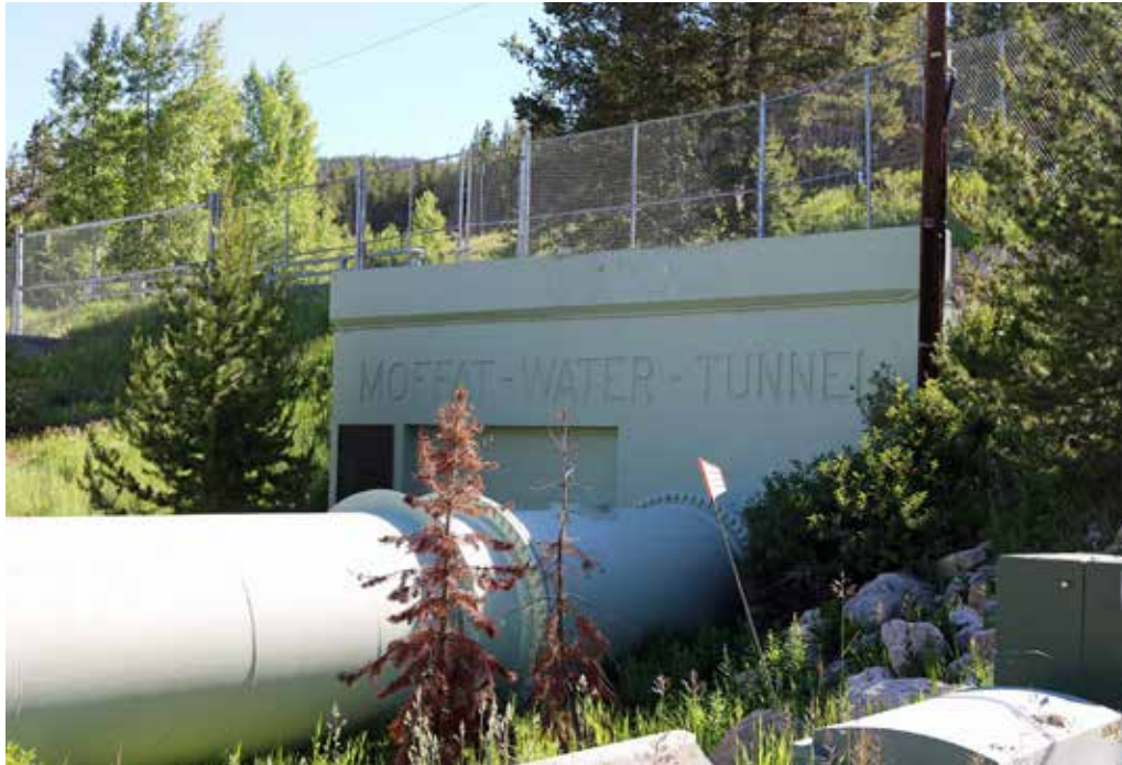
The west portal of the Moffat Water Tunnel in Winter Park, Colorado. JEFFREY BEALL
