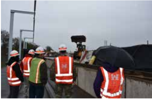
New York District Commander Mathew Luzzatto touring the Maywood Chemical Superfund Site and watching soil being placed into a railcar.
