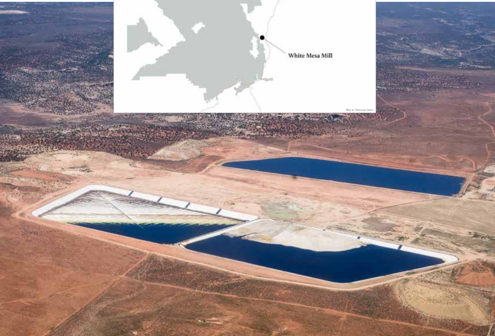
On December 2, 2021, the EPA found that the White Mesa Mill had significant amounts of radioactive wastes sitting in its waste pits that were not covered with liquid (as required by EPA rules). The EPA estimated that these uncovered wastes were emitting 10 times more radon—a cancer-causing gas—than covered material. The EPA called this violation “egregious” and deemed the mill “unacceptable for the receipt of off-site wastes” from Superfund sites, EPA’s list of contaminated places that are badly polluted and prioritized for cleanup. The EPA barred the mill from accepting Superfund waste, but did not stop the mill from accepting waste from other locations. This August 2021 photo shows the waste pits not adequately covered with liquid. BRUCE GORDON, ECOFLIGHT
